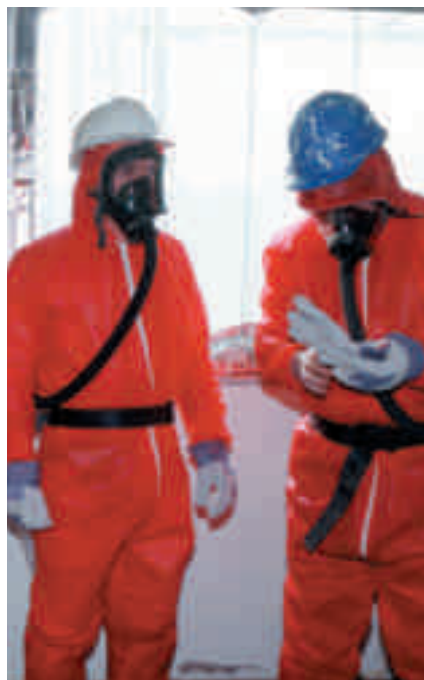
Preparing to remove asbestos
