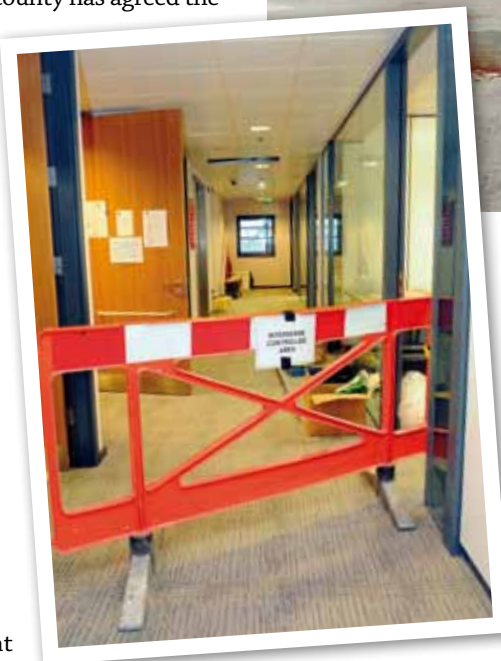
Parts of the new regional control centre are now out of bounds for repairs
