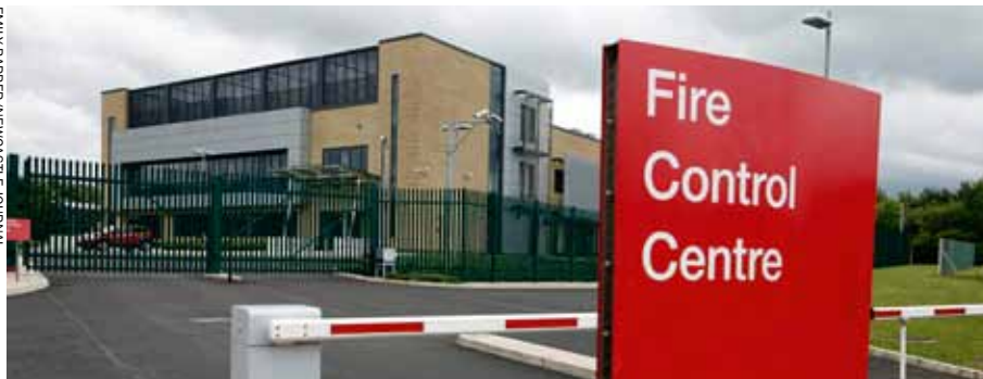
Empty but expensive: The North East regional Fire Control Centre in Durham
