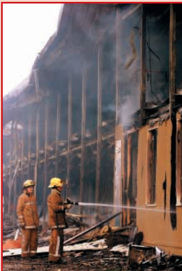
Arson attack on Yarl'swood Detention Centre – 2003
