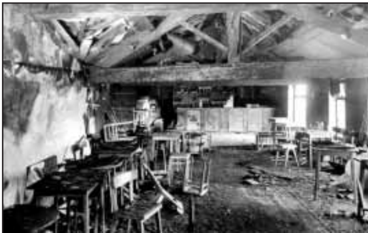
Top Storey Club fire 1961
